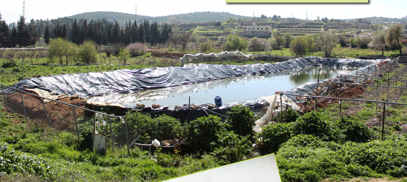
Hebron – Beit Ummar: The occupation notifies a pool with a storage capacity of 1000 m 3 and provide water for 20 dunums - February 20 th 2018
