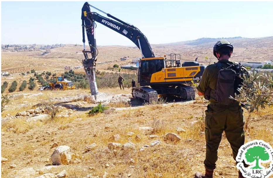
Hebron governorate – Aj-Juwaya / Yatta : during demolition of agricultural cistern – August 2024
